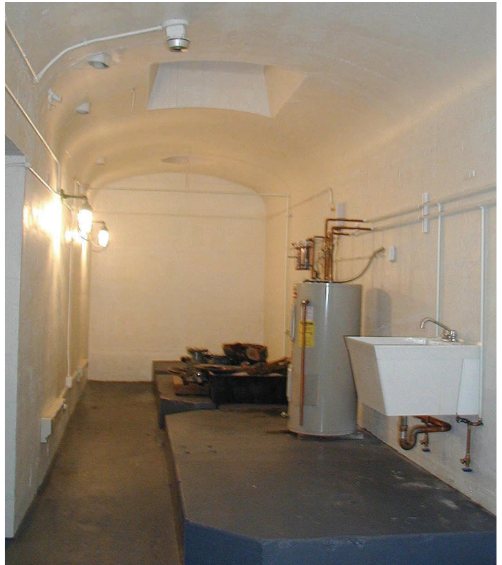
Former Fuel Storage Area in Machinery Room With New Water Treatment System Installed
