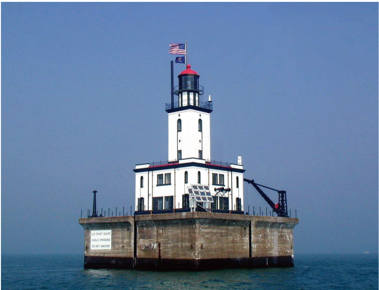
DRL as Restored, September 4, 2004
