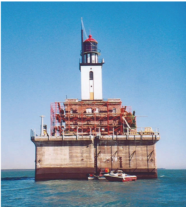
Lower Tower being Prepared for Painting
