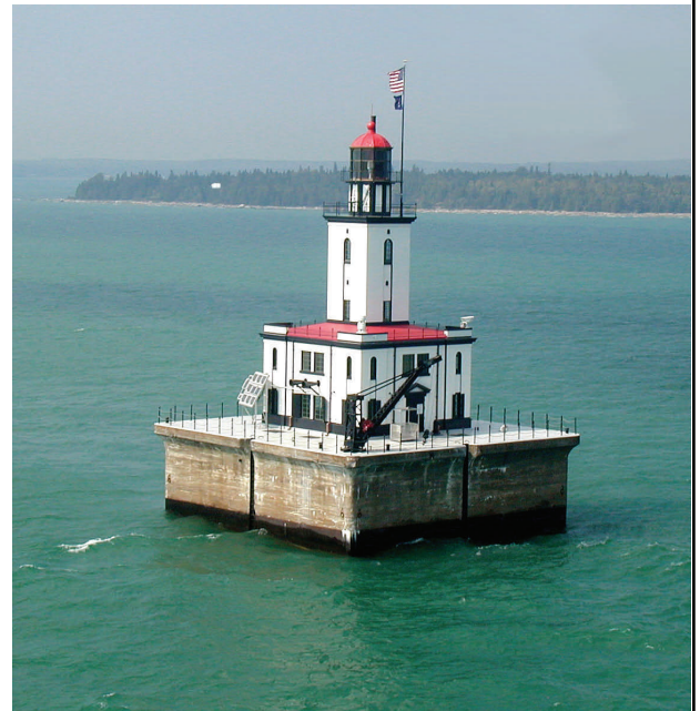
DeTour Reef Light with DeTour Point in Background (note white roof of 1861 Keepers quarters on shore)
