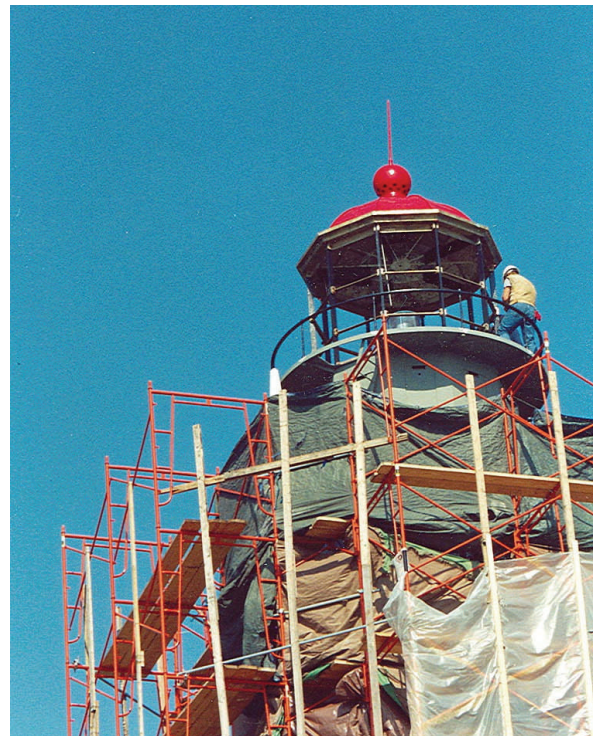
Sand Blasting Shroud Around Upper Tower
